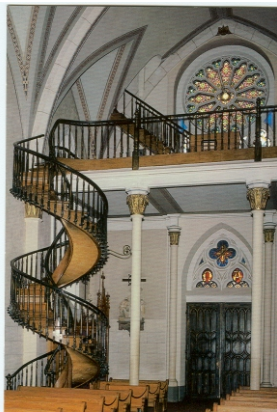
BANISTER, HANDRAILS ADDED
